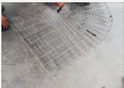
FREE-FORM BEND CUT ON SITE
