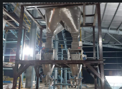
WEIGH HOPPERS AND STRUCTURE
